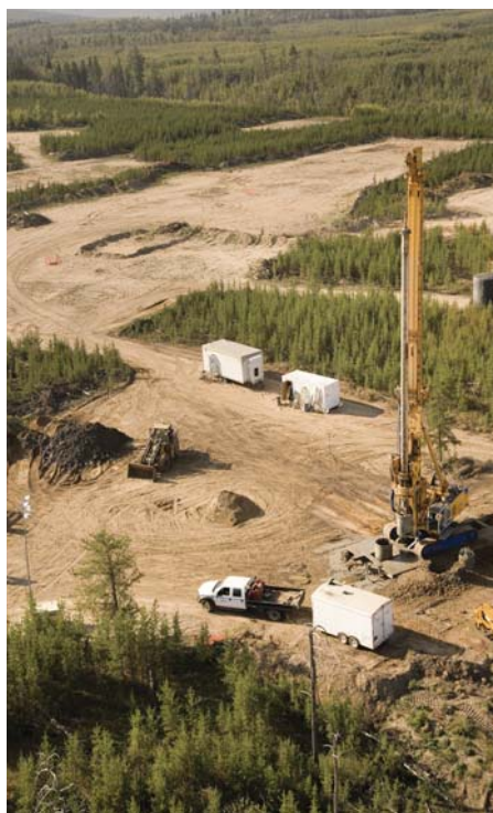
Large diameter drill
